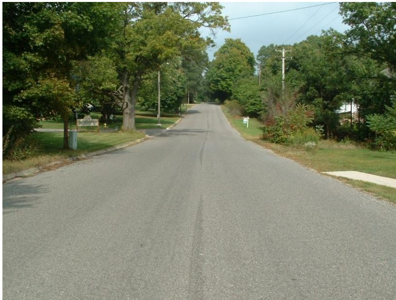
8 th Street north of Stadium Drive Crack/Chip Seal – Oshtemo Township
